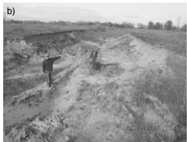
Figure 10. (a) Photo of Fremont Weir leading to Yolo Bypass after the 2004 flood season. Lag deposits are visible on the drop structure (Zone 2), and the upstream portion of the hydraulic shadow (Zone 3) is shown. (b) Headward erosion of prior sediment deposits at the downstream end of Zone 3 (hydraulic shadow) within Yolo Bypass. The view is upstream (north) toward Fremont Weir.
