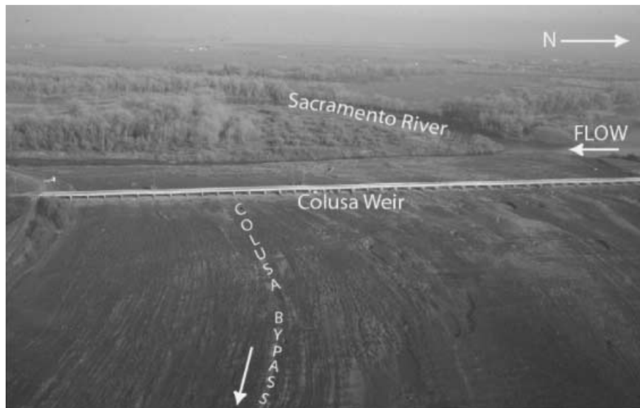
Figure 1. Oblique aerial photograph over Colusa Weir and Colusa Bypass with the Sacramento River in the background. During floods stage rises in the Sacramento until flow overtops the concrete weir (under the bridge) and moves east (down in the photo) into the bypass system. The flow first enters Colusa Bypass, then Butte Basin, before entering Sutter Bypass (not shown).
